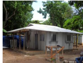
Single family home (Petit Goave) we wish to build (GPSI panel system, unfinished)
