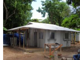
Single family home (Petit Goave) we wish to build (GPSI panel system, unfinished)
