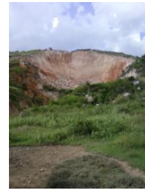
When it rains, this cavern fills up and floods the camp
